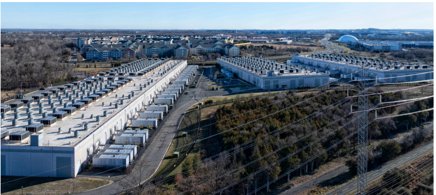
Data Center in Ashburn, Virginia.
